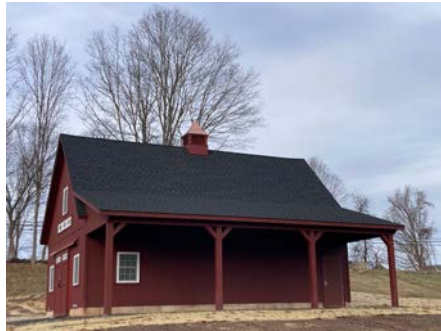
New Rocky Hill Community Farm barn at the former Straska Farm
